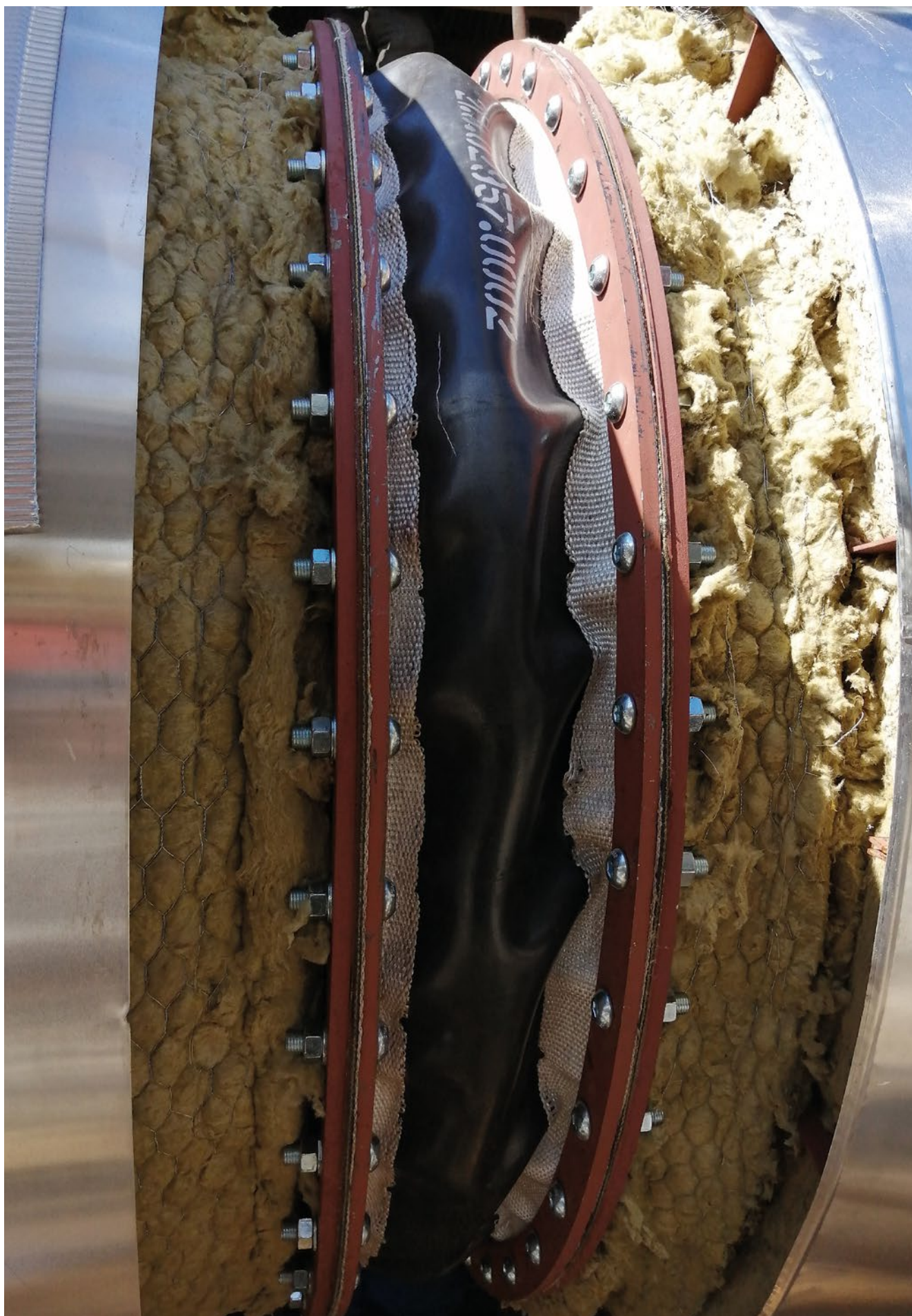
Supply and replacement of a rubber expansion joint
