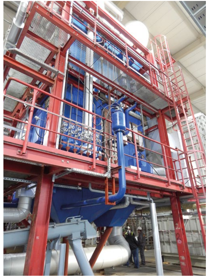
Supply and installation of shock wave generator
