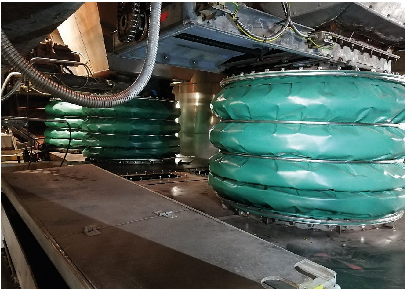
Supply and installation of a fabric expansion joint
