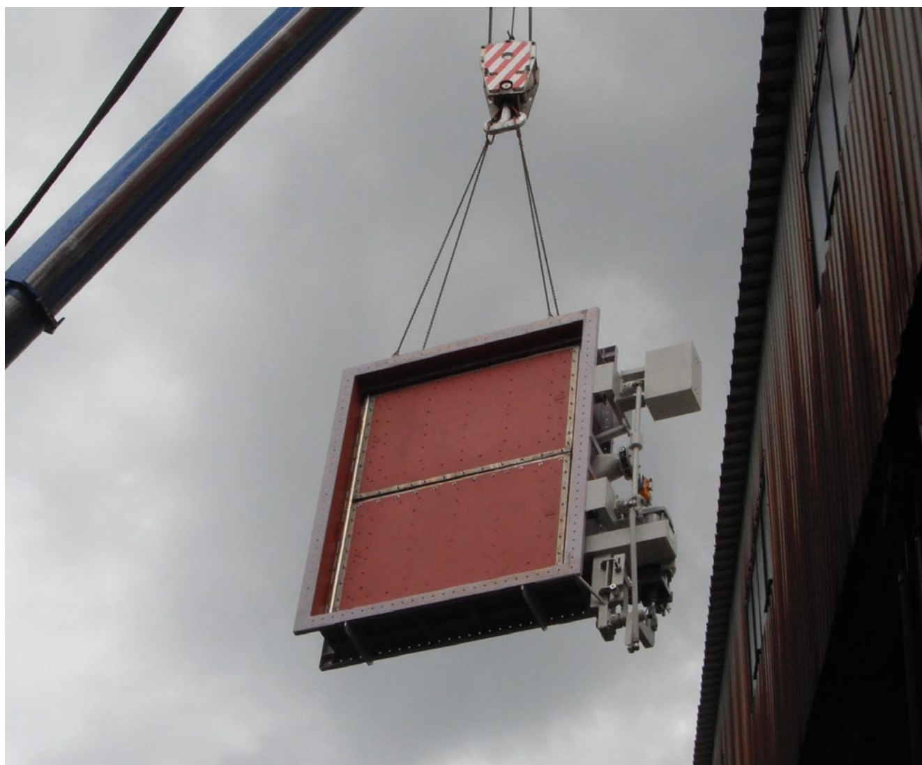
Supply and installation of dampers
