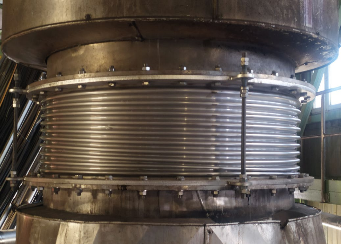
Supply and replacement of a metal expansion joint, including metal flanges
