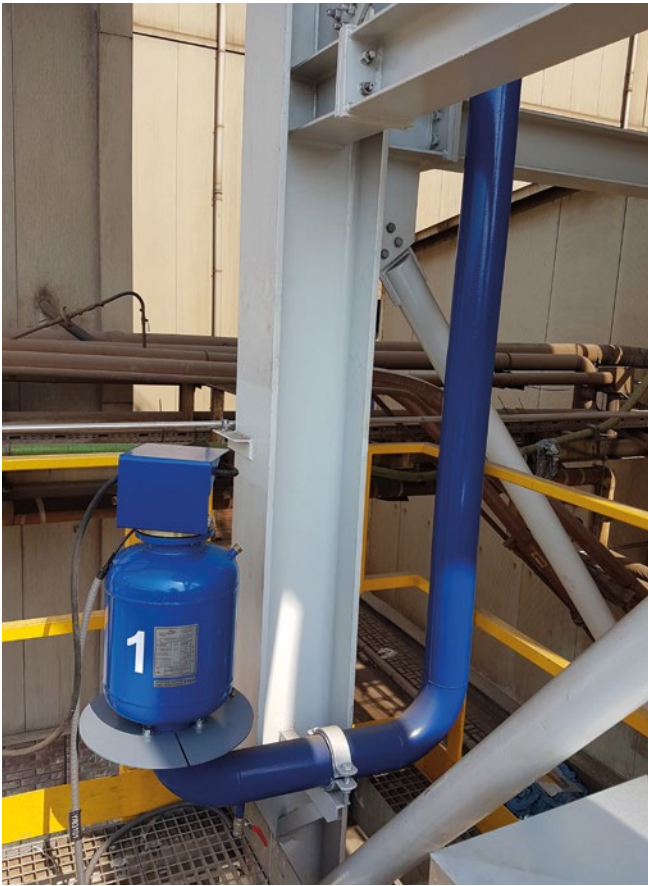
Supply and installation of shock wave generator
