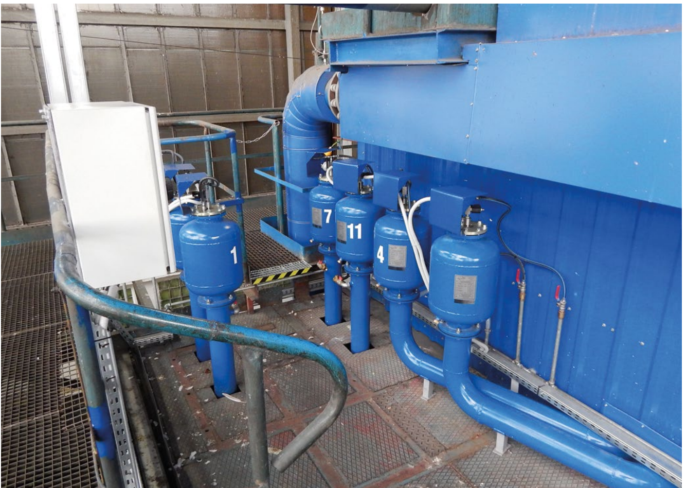
Supply and installation of shock wave generator
