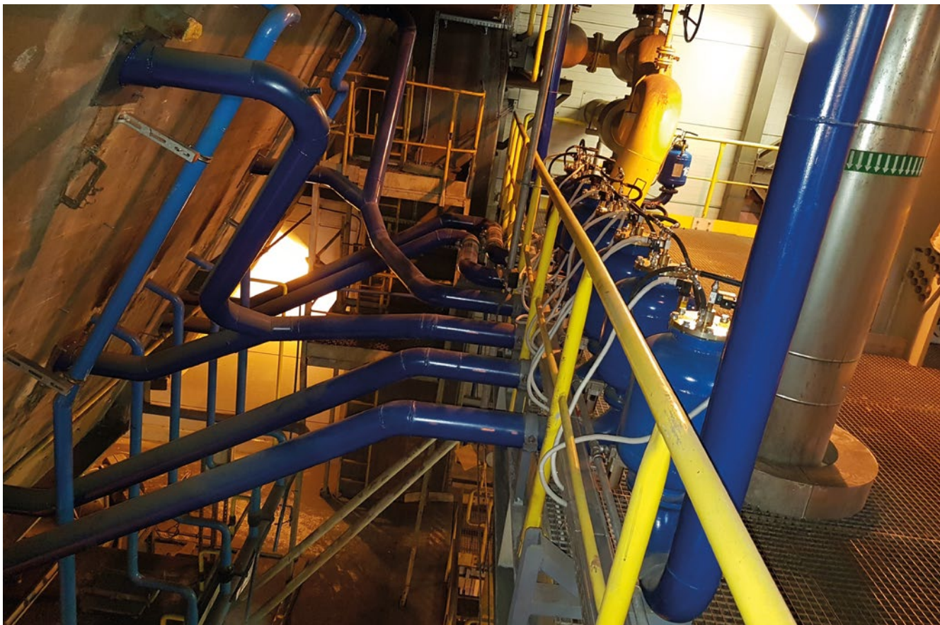
Installation of shock wave generator
